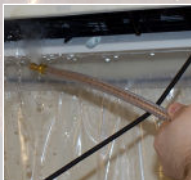
Clean fan blades and blower wheel
